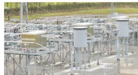
**Static Var Compensation (SVC)**, steady-state and dynamic voltage control of power distribution & transmission systems
